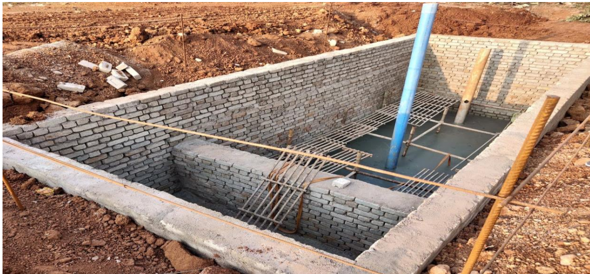
Fig. 2 Artificial Ground Water Recharging Pit under construction.
